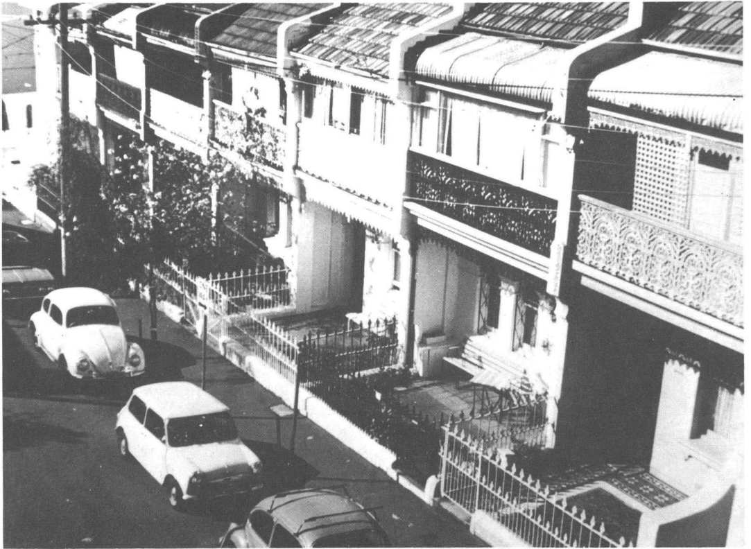
Australian terrace houses with semi-private front yards (Paddington, Sydney)
